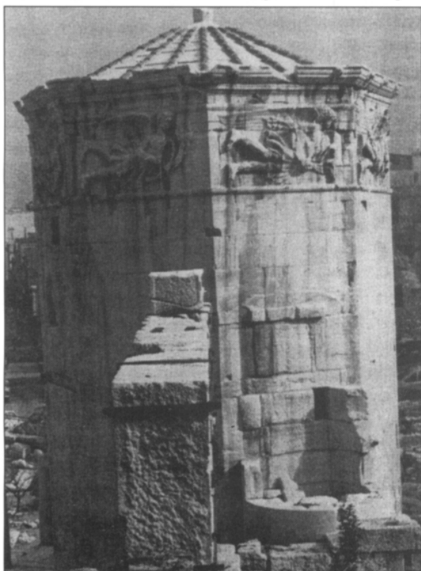
Fig. 3 South wall of Tower of the Winds, showing ruin of cylindrical annex near the base (Photo: C.K. Aked)
