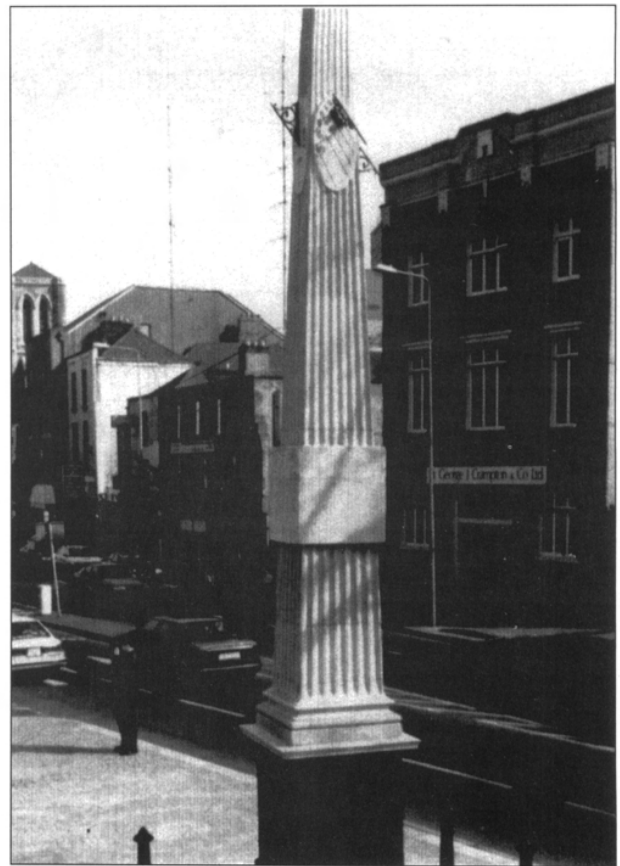
Fig. 8 The Fountain, St James's Street, Dublin: Vertical declining polyhedral pillar dial, c17th c. (Redelineation)
