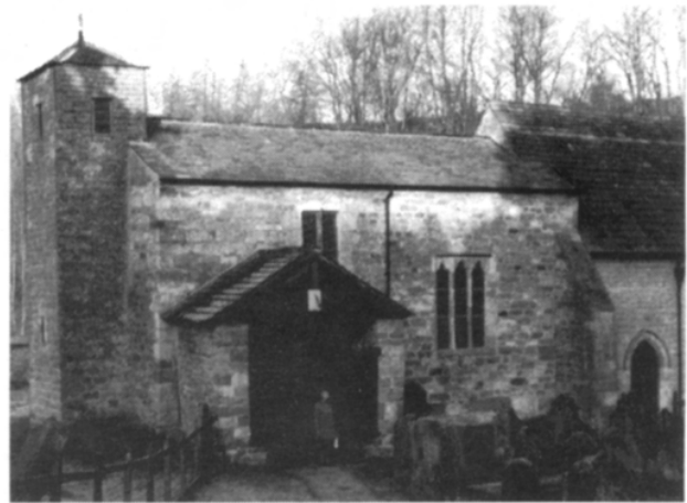
FIGURE 5: St. Gregory's Minster photographed late afternoon January 1992, with hard frost on the ground
