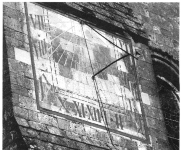
FIGURE 6: The rather crude gnomon of the Chichester Cathedral sundial.
