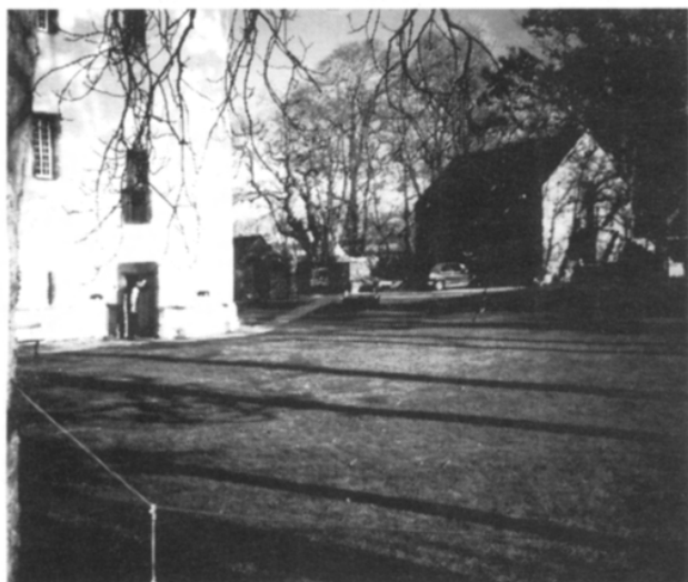
Figure 5: Kinkell Castle, Studio and Foundry
