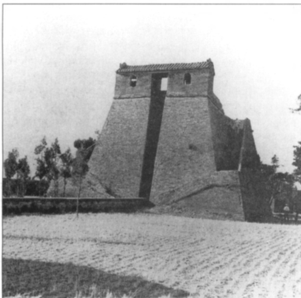
FIGURE 7: The 'Tower of Chou Kung' at Gaocheng, some 50 miles SE of Luoyang, north-central China. (After Needham 20 .) The horizontal iron bar constituting the gnomon had not been restored when this photograph was taken.
