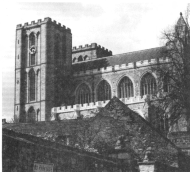
FIGURE 7: Part of Ripon Cathedral showing some of the newly restored stonework.
