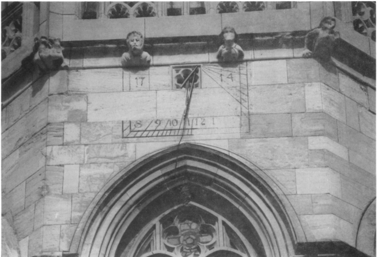
FIGURE 6: One of the dials delineated by the St George's Chapel, Windsor, in 1714. 270 years have almost effaced it. Note that the lower left part is on a better piece of stone, also how most of the gargoyles have deteriorated.
