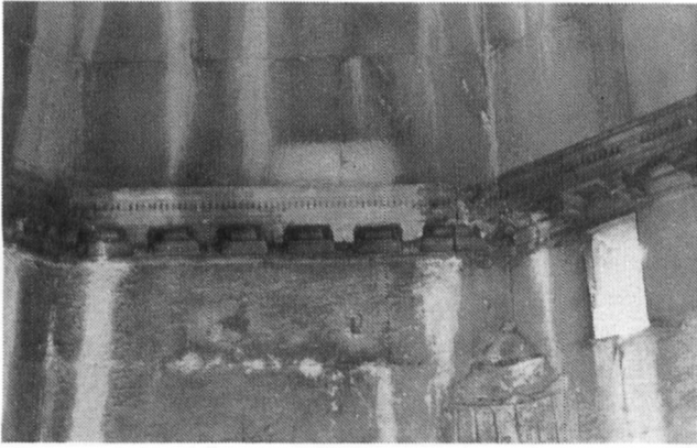
FIGURE 6 Part of the interior roof of the Tower of the Winds, showing one of the holes cut in the wall to admit light.
