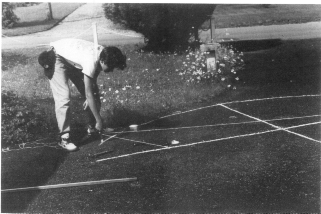
2: Marking our the playground dial using the well known method for drawing an ellipse.
