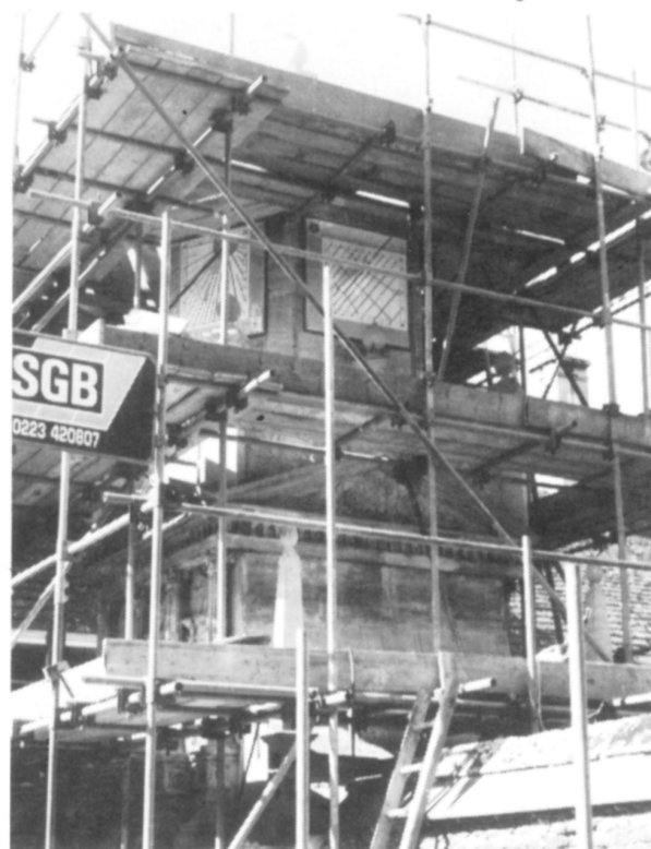
3. THE GATE OF HONOUR, CAIUS COLLEGE, SCAFFOLDED FOR RENOVATION.
