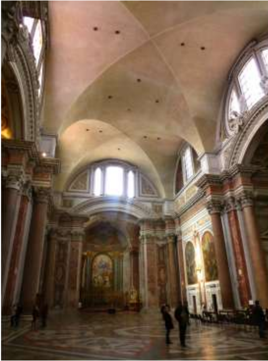
Fig. 1. Looking towards the northwest transept of Santa Maria degli Angeli e dei Martiri, Rome. The 30-metre high vaulted ceiling is a remarkable remnant of the original Diocletian baths of AD 306. Photo: Sullivan.
