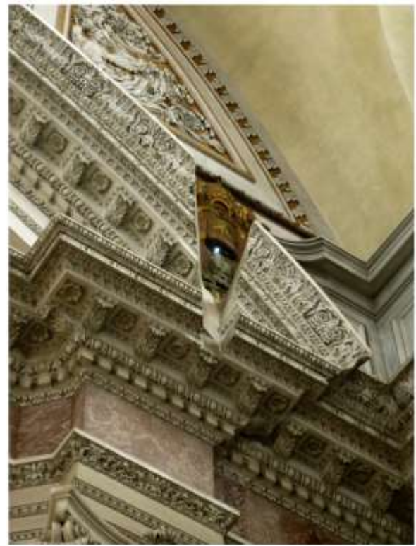
Fig. 5. The southern aperture. A major revision of the basilica interior in the mid-18th century introduced an architrave, complete with its accommodating cutout section. Light from the sky can just be seen through the aperture (diameter about 2–4 cm). Photo: Sullivan.
