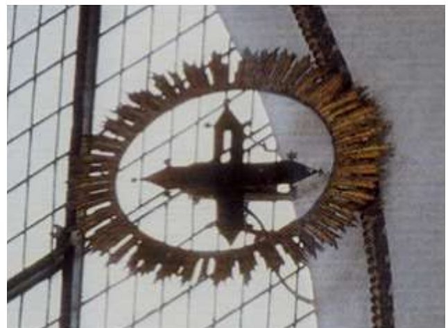
Fig. 17. The aperture for the North Celestial Pole and Polaris. The centre of the vertical slot is about 24.4 metres above the basilica floor and 0.91 metres to the west of the meridian line. See Fig. 6. Photo: Catamo and Lucarini. 1
