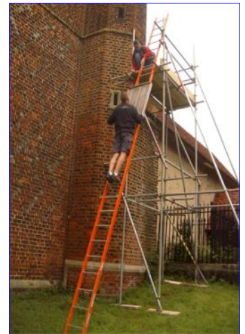
Fig. 3. Removing the old dial from the tower.
