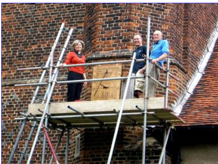
Fig. 13. The newly-installed dial.
