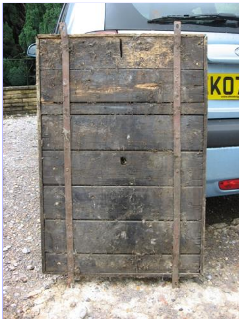
Fig. 4. The construction of the back of the old dial.
